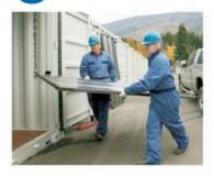
Position panels in desired location within the container. Line each half up with each other across the container.
